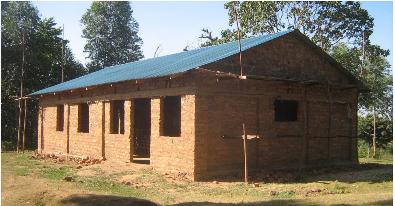
Mercy Children's Academy in January of 2011. Construction is ongoing.
